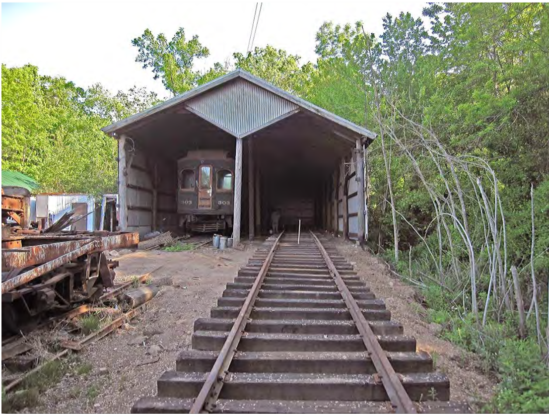
Relayed Track #2 at the Northern Barn on May 22, 2015.
