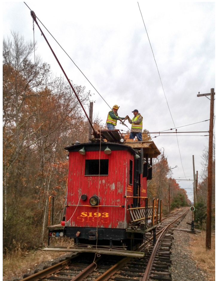
Ray Nobile & Bill Stoba removing the failed wire frog at the west end of Newberry Siding
