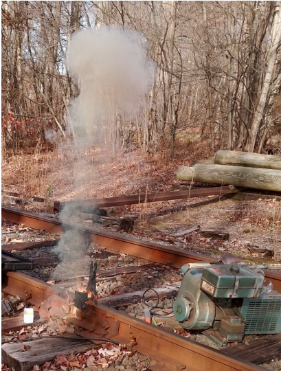
Signal bond replacement at Winkler Rd on December 16, 2017
