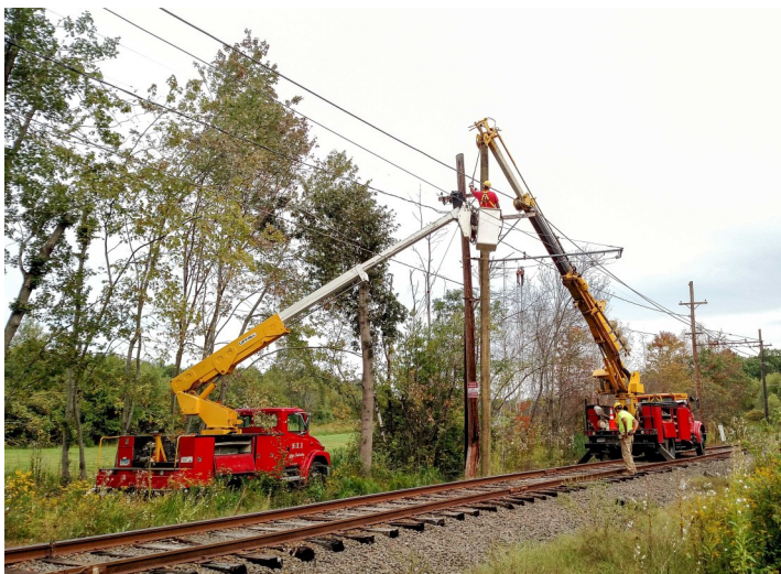
Contractors replacing a damaged pole east of Winkler Rd.
