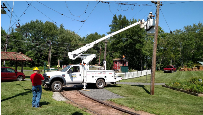
Wire Frog Repairs with S-193 and BT-1
