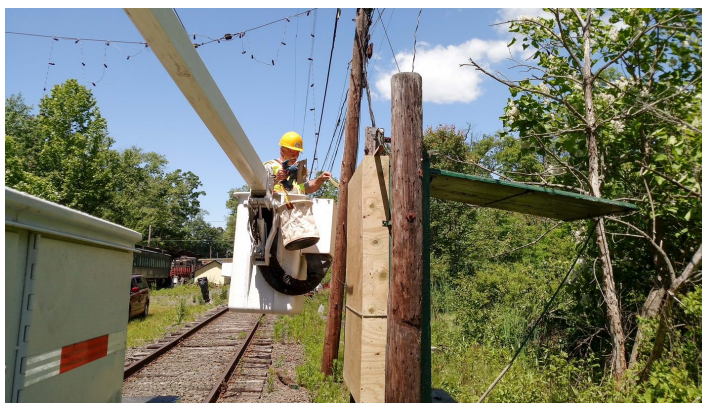
Signal Case Repairs being made
