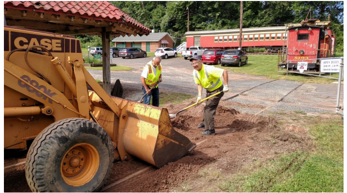
Clearing Dirt along North Road 1 for Operations
