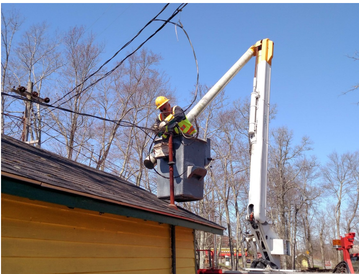
Line Shop Power Drop Repaired
