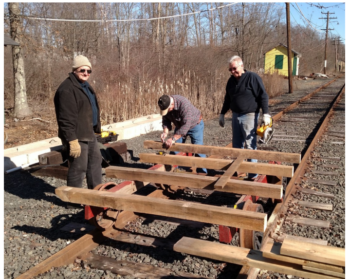
Flat Car being rebuilt by SC&ET Department Volunteers
