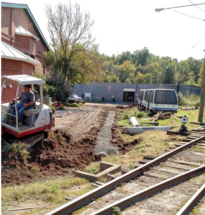
Visitor Center Drainage Work being completed
