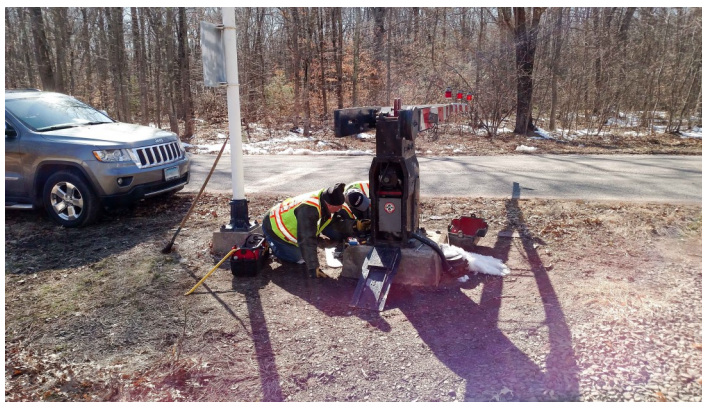
Borrupt Road Gate Repairs
