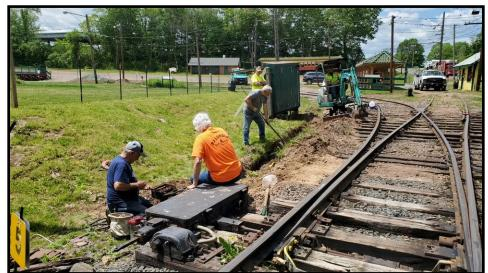
With the completion of the rebuild of #2 Track at North Road Station, track circuit wiring as well as the cable from the North Road Signal case to the North Road Switch mechanism were replaced enabling the return of remote operation of the North Road Switch to North Road Station.
